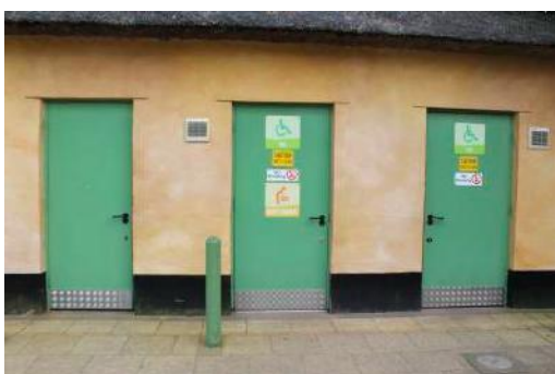
Disabled toilet entrance
